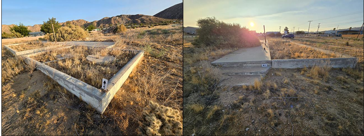
Figure 8. Concrete foundation within the project area. Left : view to the northwest; right : front steps, eastern view. (Photographs taken on August 24, 2024)
