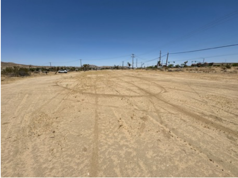
Photo 7. View of recently disturbed area with fresh blade marks in the central project site, facing northeast. June 17, 2025.
