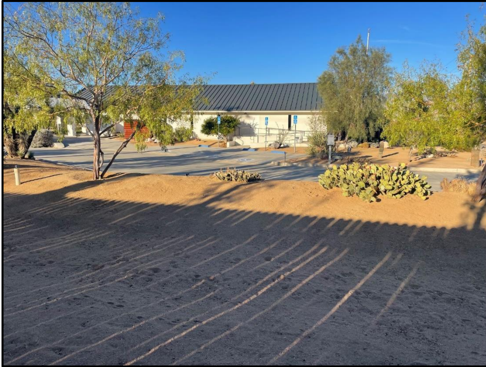
Plate 4.2-3: Overview of APN 0588-021-21 from the eastern boundary, facing west.
