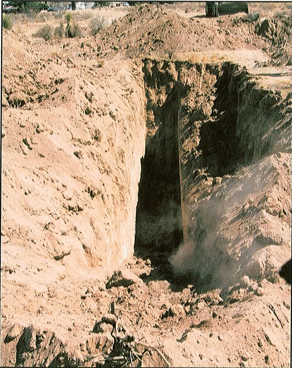
Photo 4: Fault trench No. 4 located directly to the north of Fault trench No. 2. A discernable fault trace was located within the trench.
