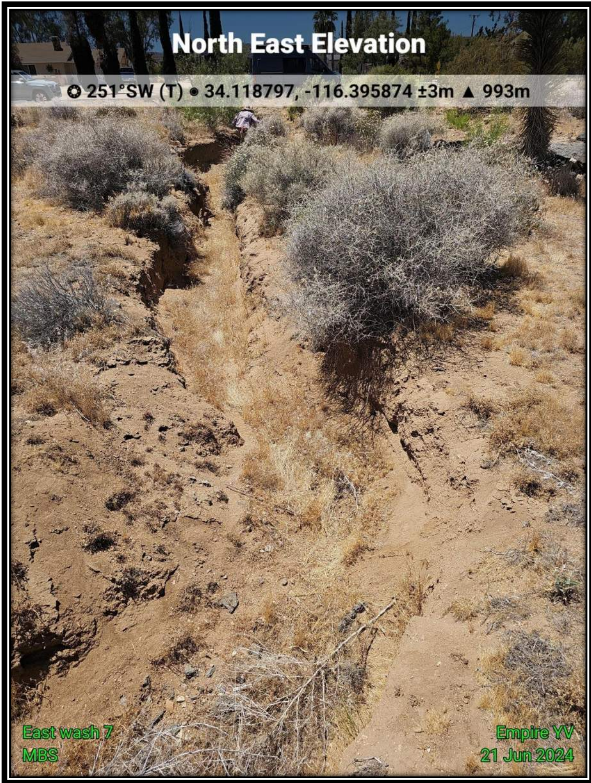
Exhibit 7E. View of the East Wash, facing southwest.
