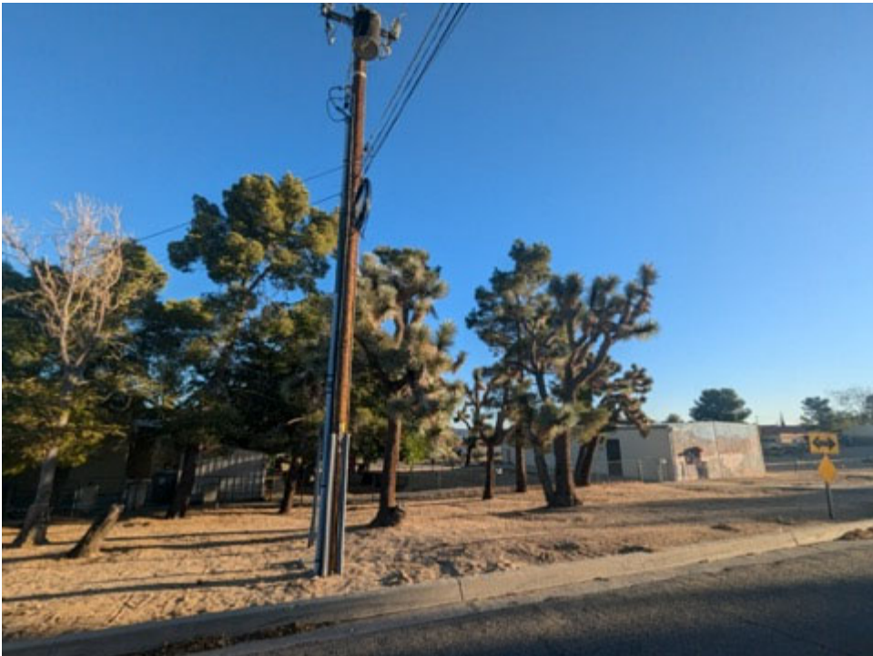
View of proposed utility line trench route facing northeast.
