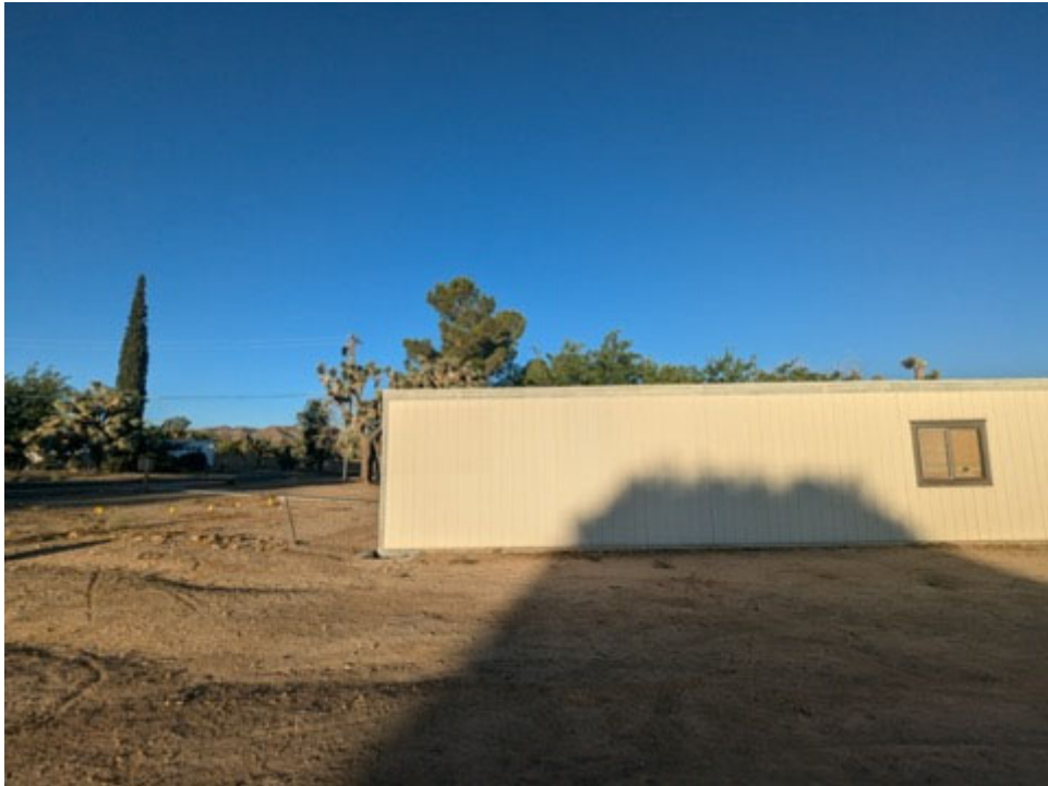
West facing view from the project site.
