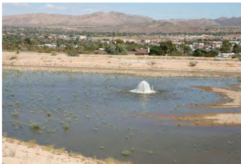
A water recharge facility.
