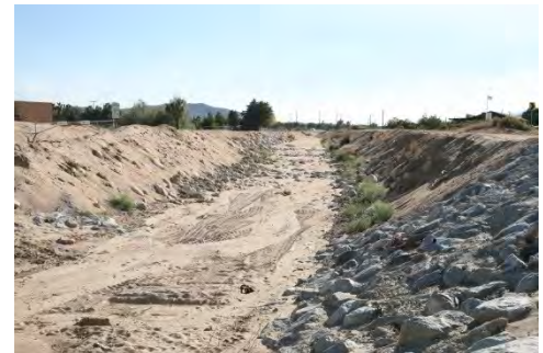
Unlined drainage channels are part of the Town's stormwater runoff management system and provide opportunities for new trail linkages.
